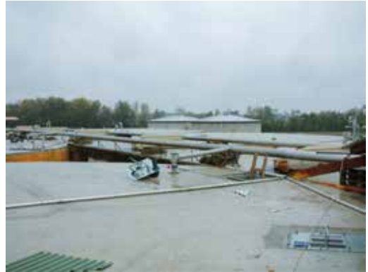
Figure III.5.3: Fermentors with rigid covers (Nyírbátor, Bátortrade Kft.)
