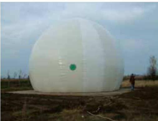
Figure III.5.7: Double-walled foil gas collector container – experimental equipment
