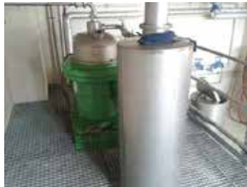
Figure II.10.17: Degreasing with separator (Photo: László Simon)
