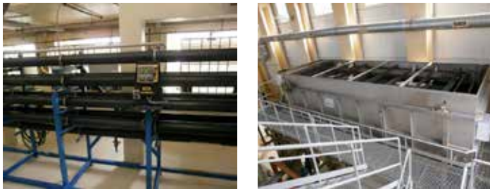
Figure II.11.13: Pipe flocculator (on the left) and flotation equipment with dissolved air (on the right) (Source: ATEV Zrt Hódmezővásárhely plant, 2014)
